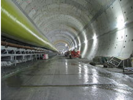
Tunnel under construction
